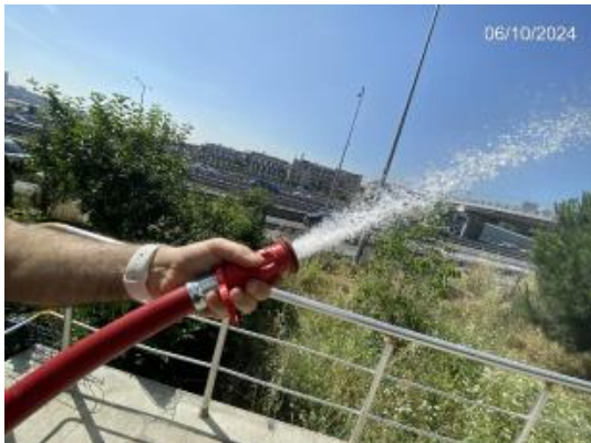
fire hose testing .JPG
