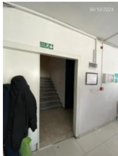
emergency exit door of the production area.JPG
